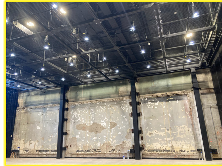
The new Victor Shargai Theatre will be Studio's home for our most innovative productions; this is the theatre's newly installed tension grid.
